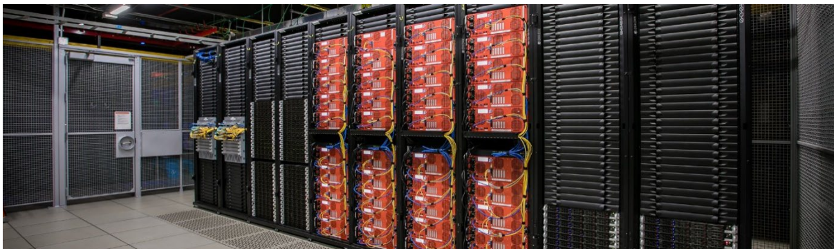
Figuur 9: veertig Netflix Open Connect Appliances (caches) in 4 volledige rekken (bron: Netflix)
