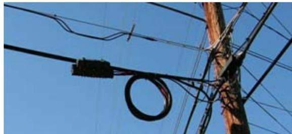
**Figure 21 Optical fibre rolled out via posts. (Source: UGent)**
