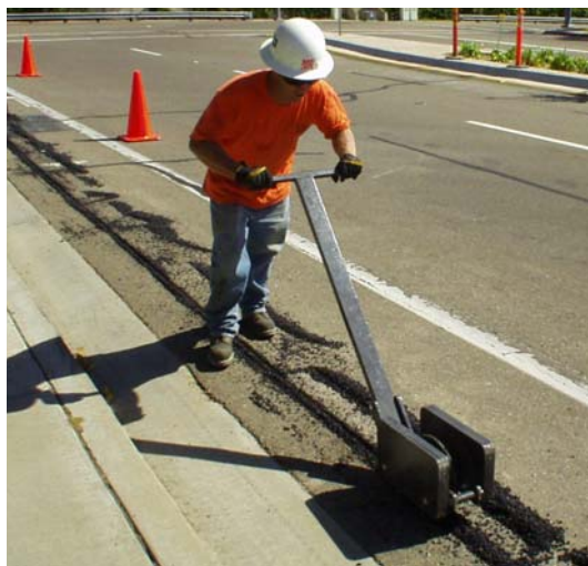
Figure 23 Micro-tranchée
